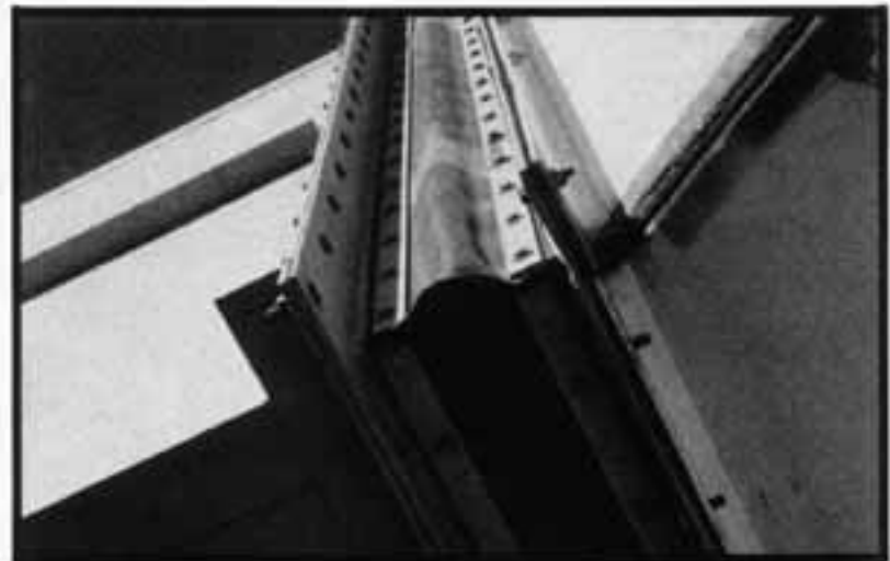
STYLE #150 NEOPRENE/NYLON REINFORCED (BLACK) DUCT EXPANSION JOINT 1/8" THICK WITH SEALED CORNER
